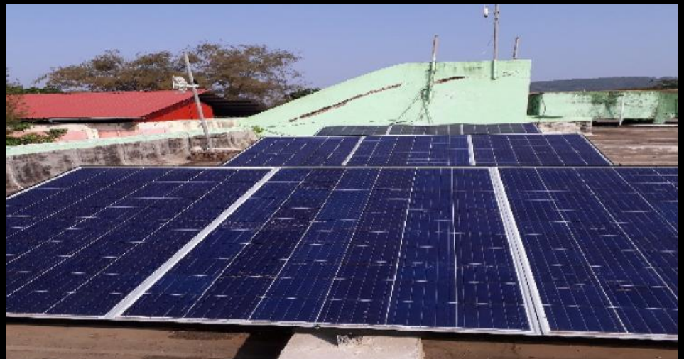
MOUNTED SOLAR PANELS
