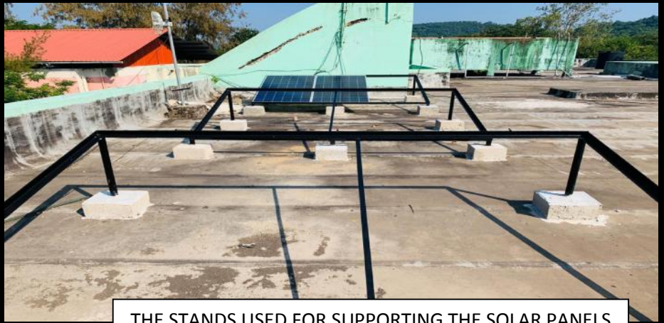
THE STANDS USED FOR SUPPORTING THE SOLAR PANELS
